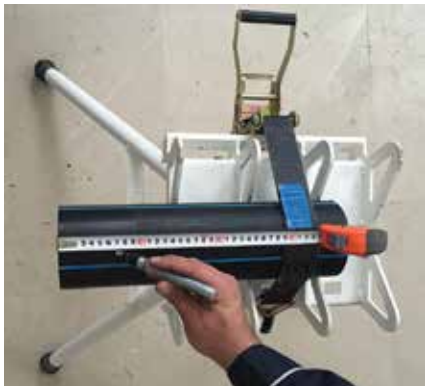
1- Measure area which has to be scraped with marker.
