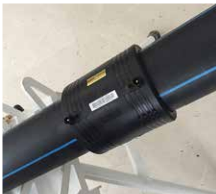
5- Place second pipe end up to first pipe, push electrofusion coupler back onto the second pipe until the second marking area with bare hands after scraping and cleaning.
