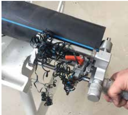
2- Scrape at last 0.2 mm of outside pipe surface to remove oxidation and other contaminants.
