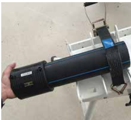
4- Insert pipe into electrofusion coupler.
